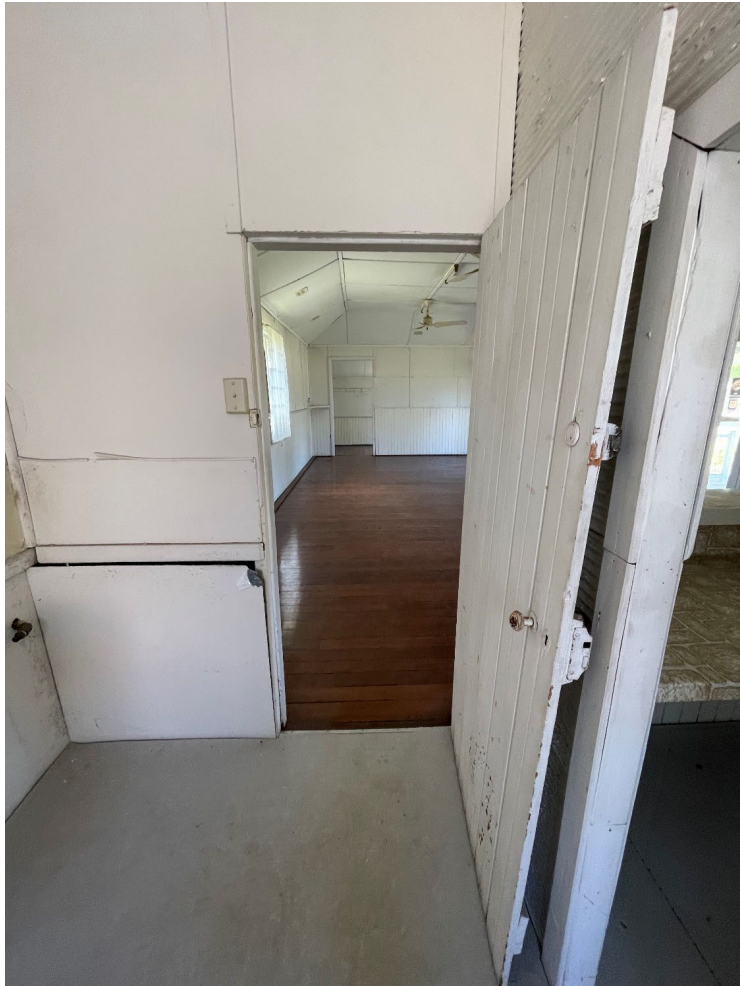
Figure 38: View to Clubroom Pavilion space from kitchen
