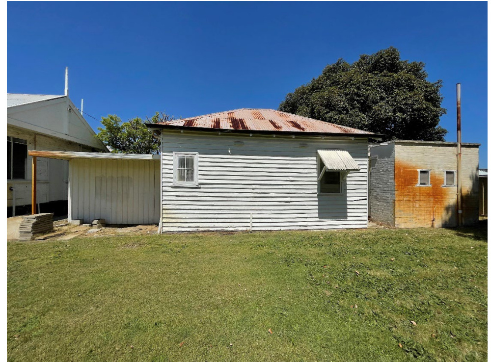
Figure 29: Rear view of Croquet Equipment Store and toilets
