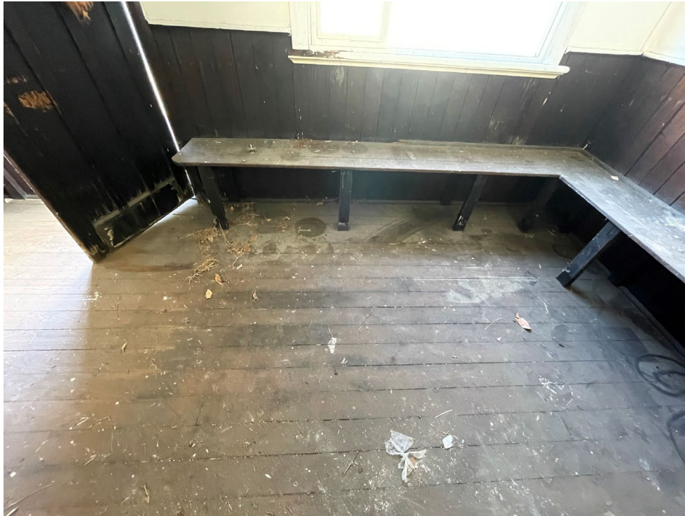
Figure 40: Croquet Equipment Store bench seating
