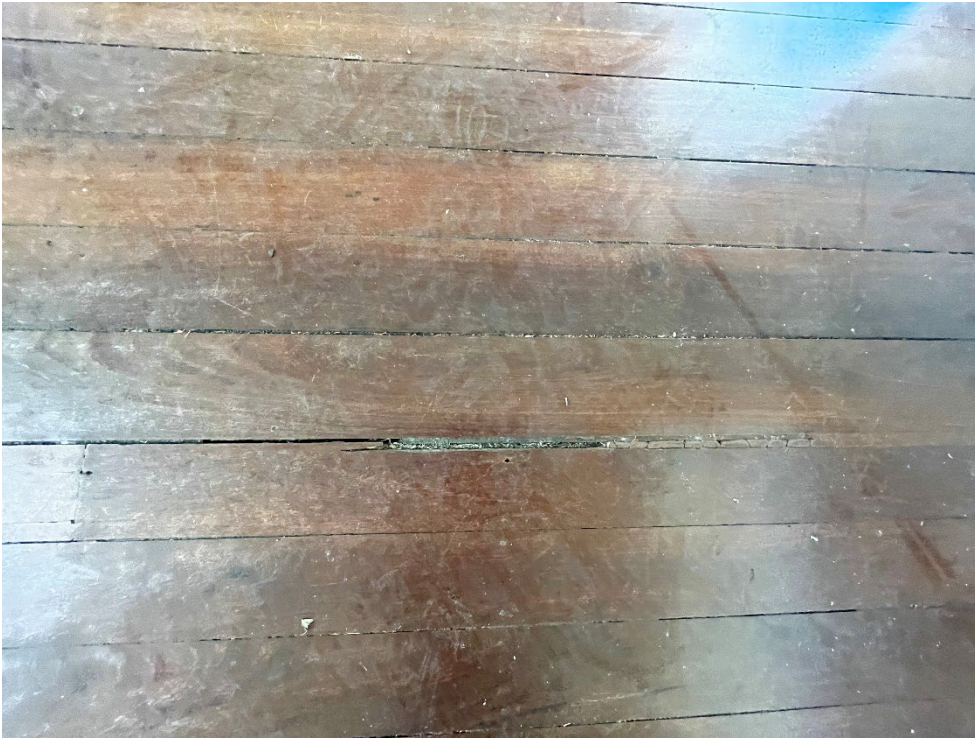
Figure 32: Clubroom Pavilion floorboards detail
