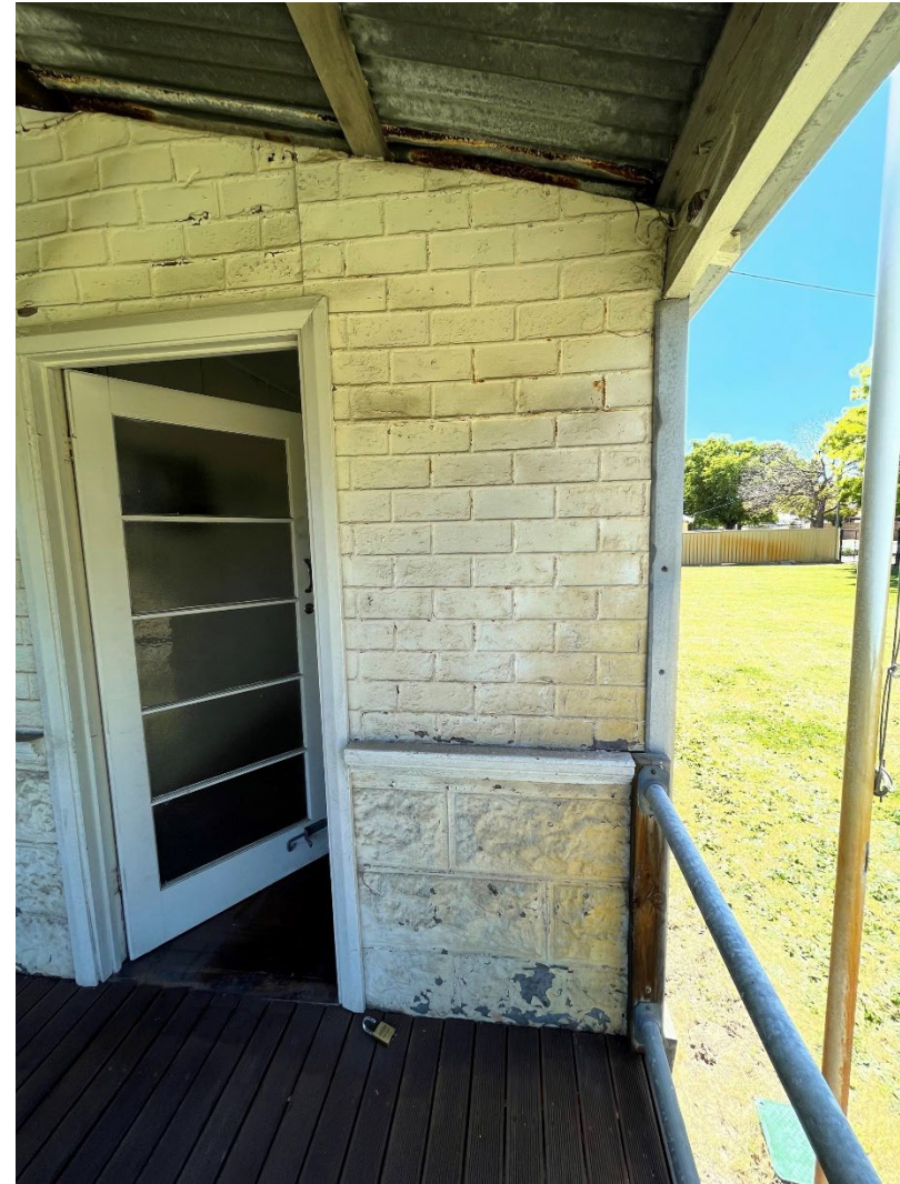
Figure 23: Pressed metal cladding on south elevation
