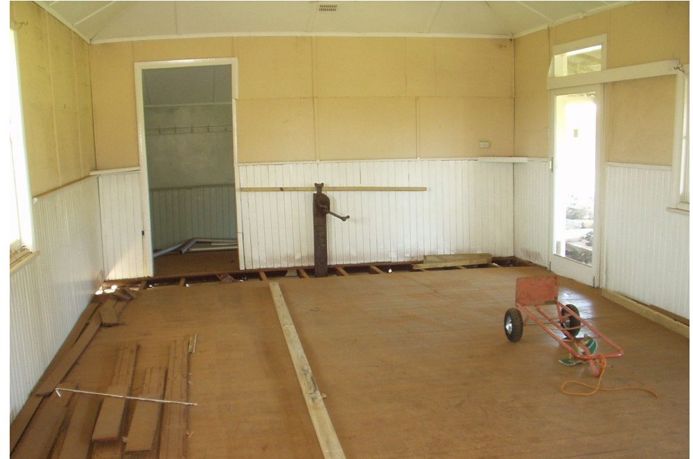
Figure 9: Internal view showing restumping works, 2006
