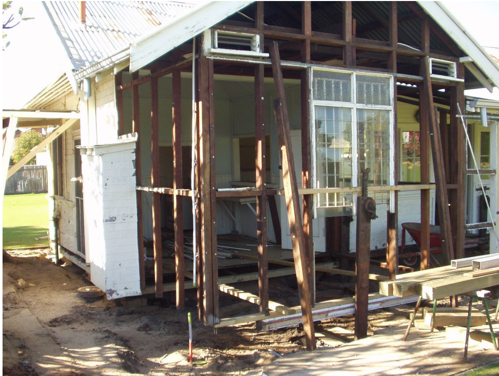
Figure 10: Recladding and restumping of servery, 2006 Courtesy Town of Victoria Park.
