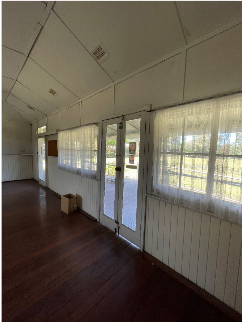
Figure 34: Glazing and roof vents
