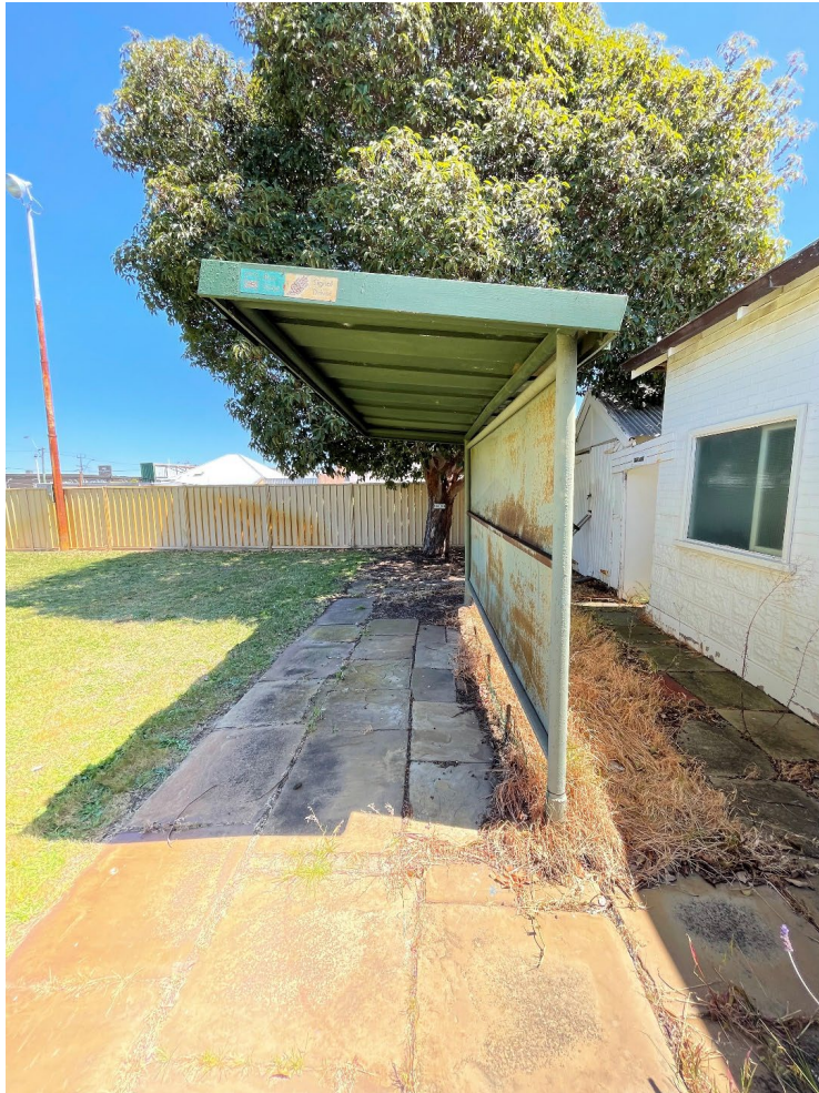
Figure 30: Relocated Bus shelter
